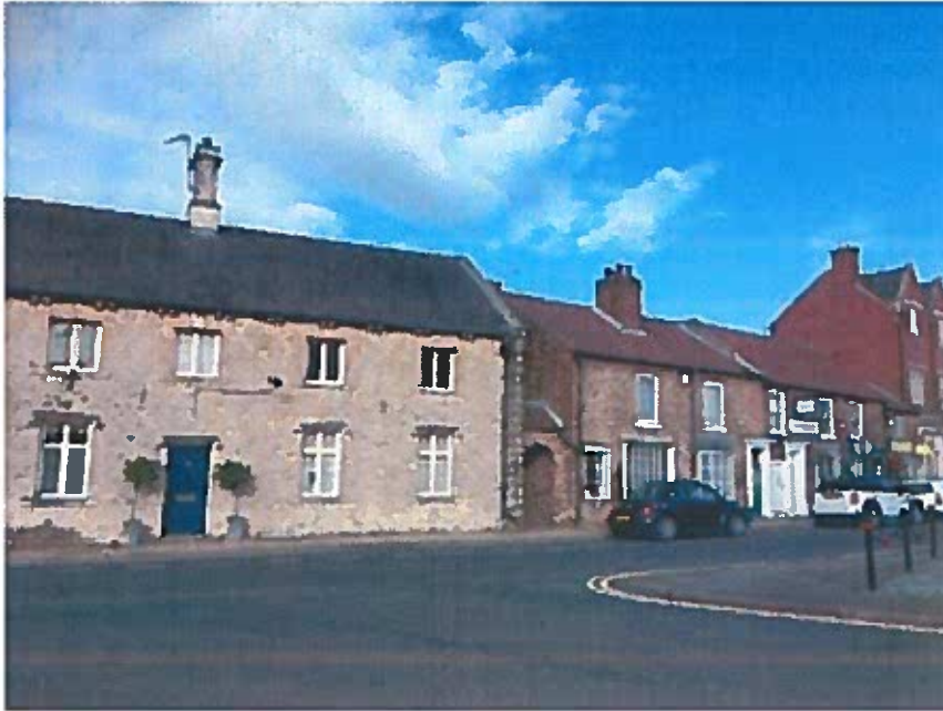
View looking to the right of the premises
